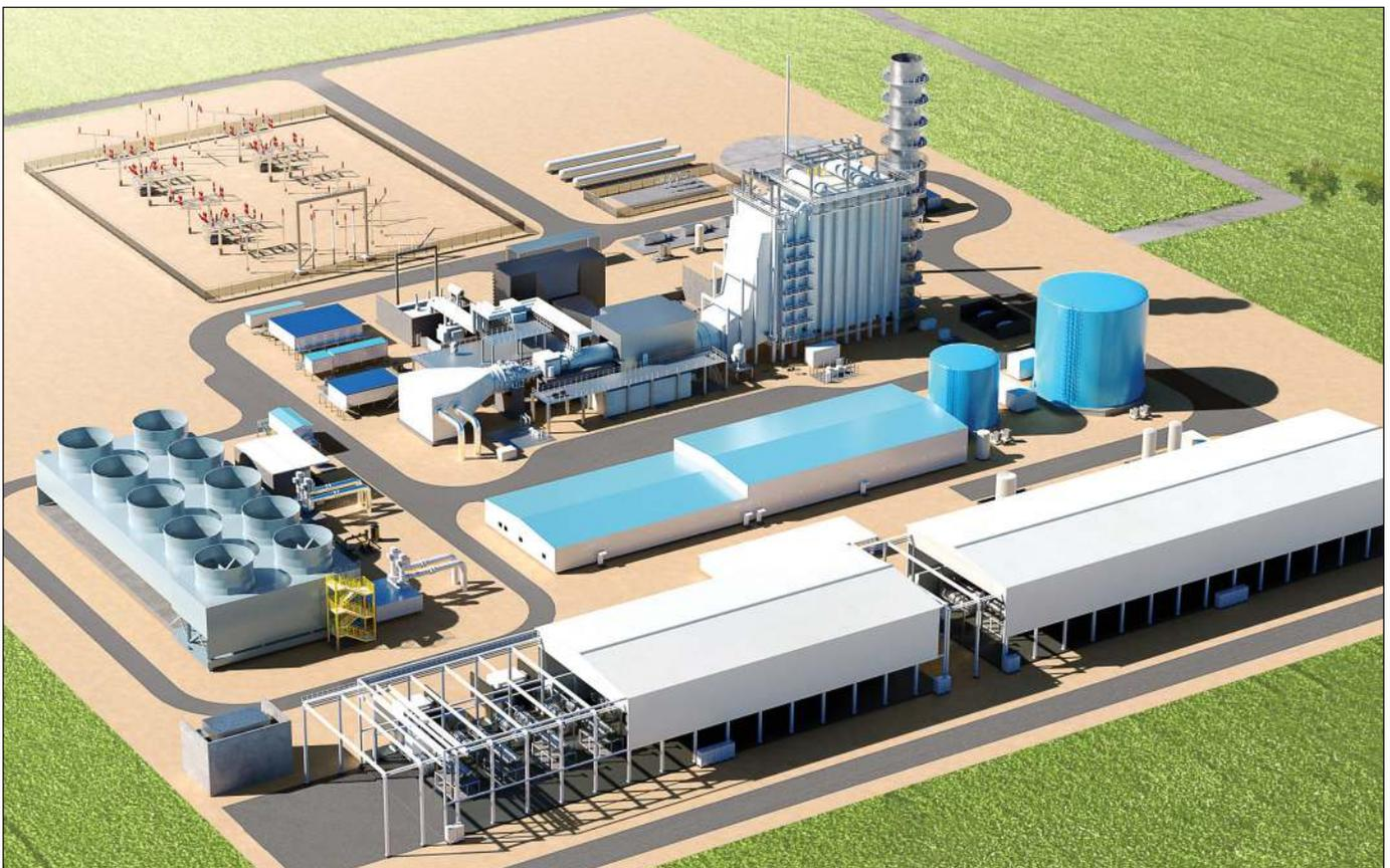
**Hydaptive integrated plant.** Conceptual plant layout designed around a single-shaft hydrogen-enabled gas turbine combined cycle unit. Site incorporates two electrolyzer buildings (foreground), air-cooled condenser (left), hydrogen storage field (background) and switchyard.
